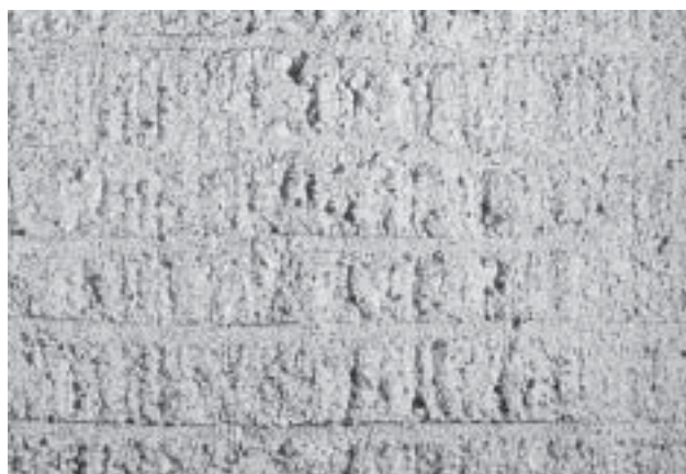
Typical hessian-drag and tynd finish
