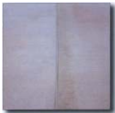
Finished G-Seal joint
