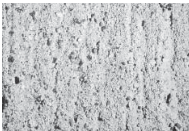
Typical hessian-drag finish
