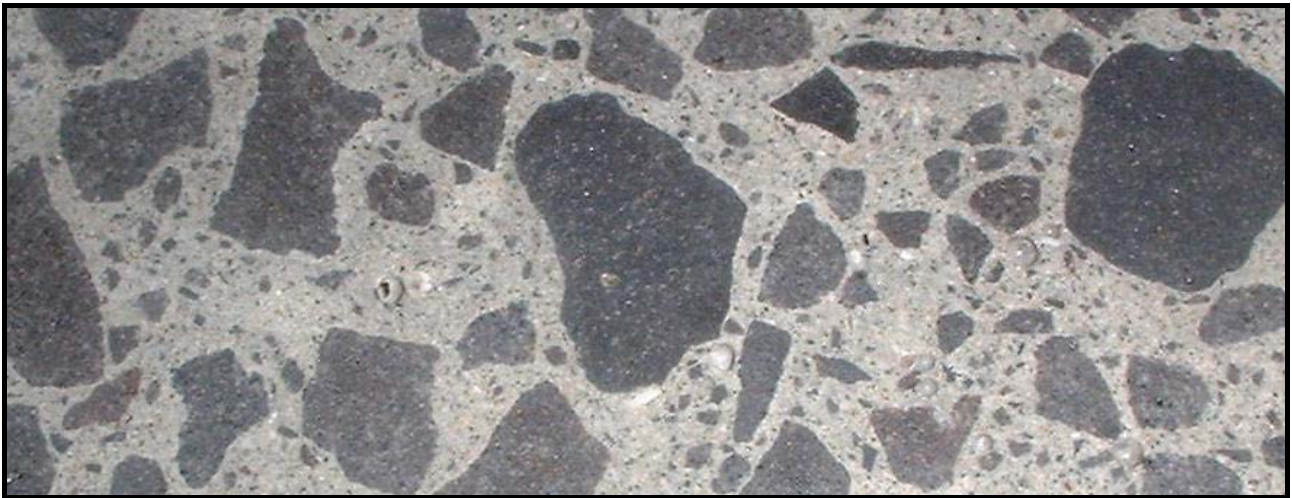
Figure 4: Concrete containing Bombay aggregates
