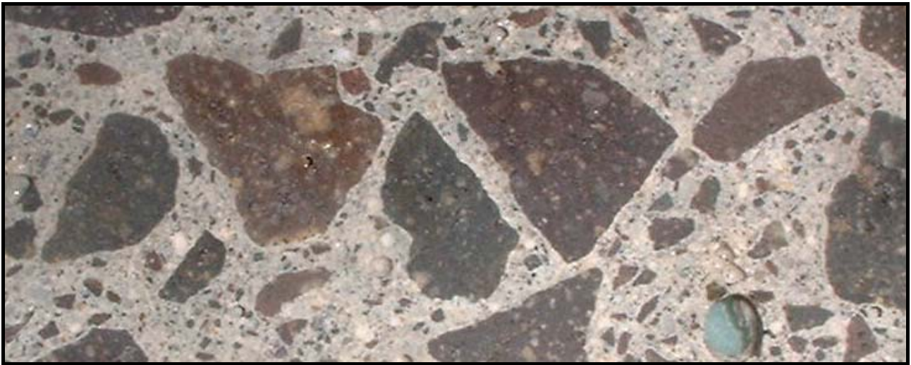
Figure 7: Concrete containing Tauranga aggregates
