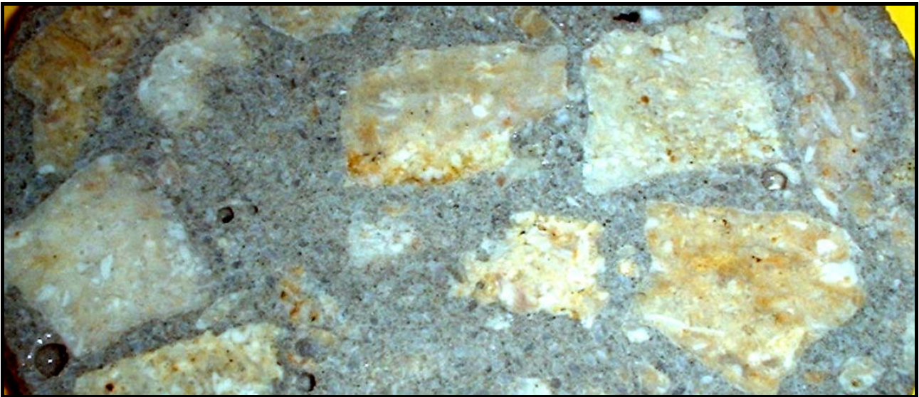
Figure 18: Concrete containing Waiau aggregates
